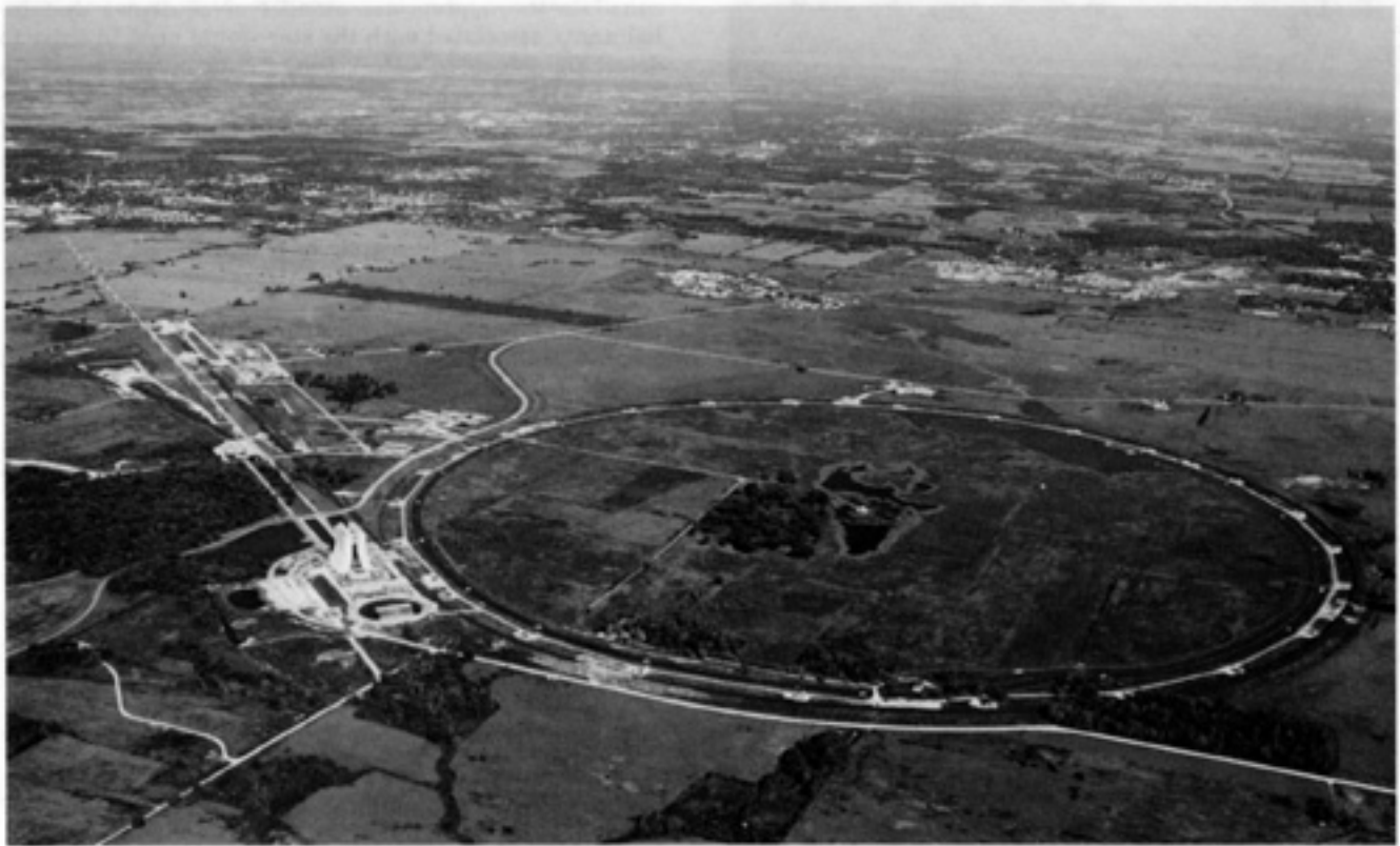
Fermilab with the 2 kilometer diameter "Main Ring" at bottom center. The main office tower is just to its left and extending diagonally up to the left are the beam paths.
