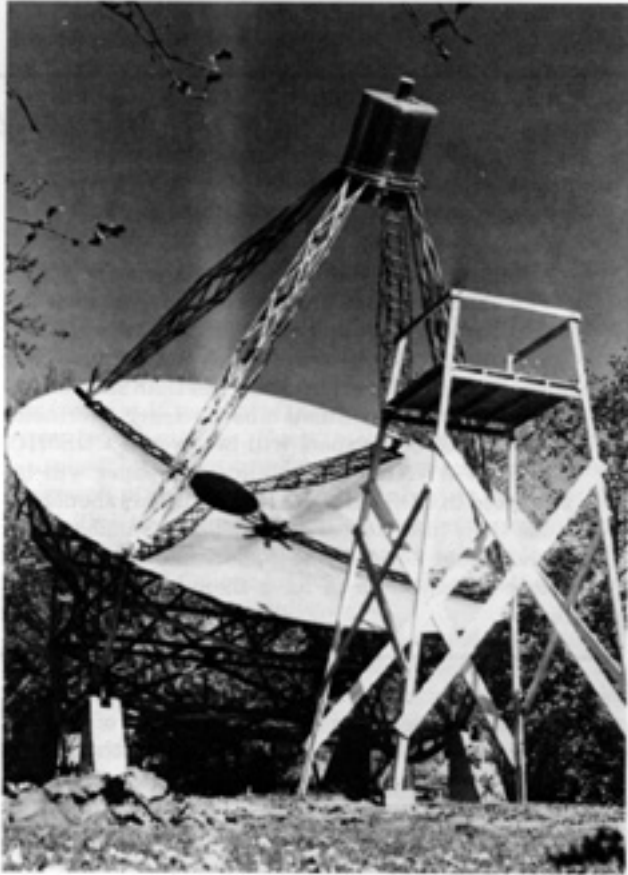
Grote Reber's dish antenna at Wheaton, Illinois, in 1938, the prototype of the modern radio telescope.
